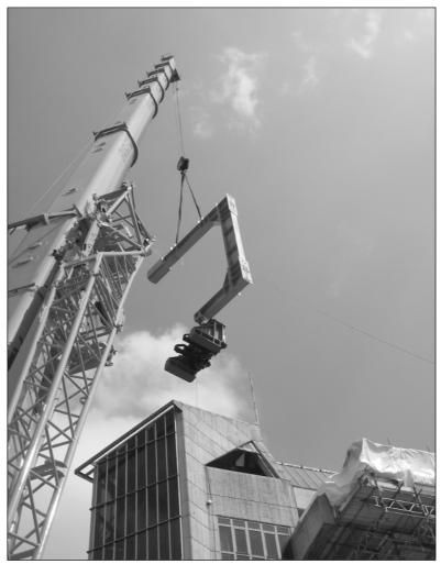
Figure 4 Lift operation using C hook
